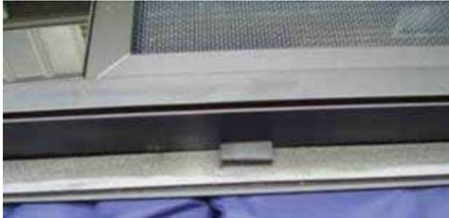
I do not know what type of shims Peninsula provides to center the window in the frame. I made shims out of hard rubber, and, by trial and error, settled on a shim height of about 3/8-inch. Note the shim is narrow so it will not impinge on the compression action of the compression frame. Once everything looks good, remove the protection film from the foam and glue the shim to the tape.
